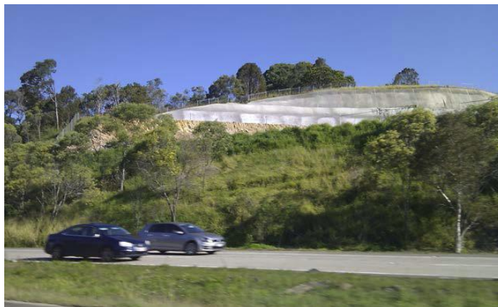
Photograph 1 – Shotcrete Retaining along the northern side of site as viewed from the Pacific Highway
